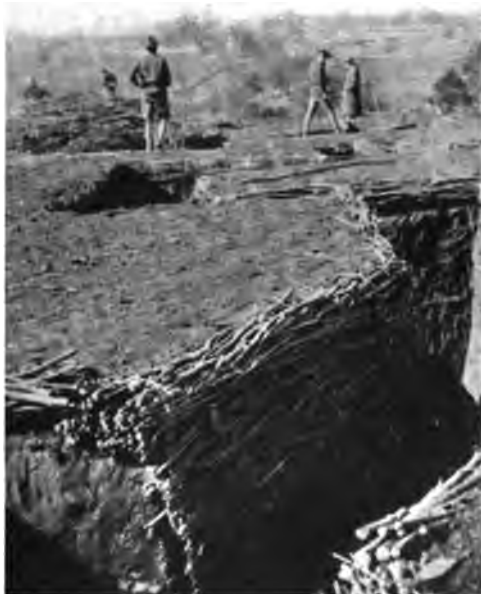
BRUSH REVETMENT—TRENCHES AT CAMP WADSWORTH
