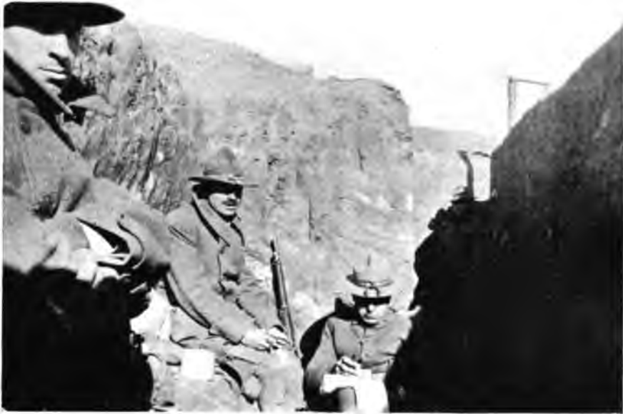
TRENCHES AT CAMP WADSWORTH
