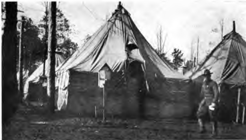
FOR THE WINTER 1917-1918, WOODEN FLOORS AND SIDES WERE BUILT INTO THE TENTS IN THIS MANNER
