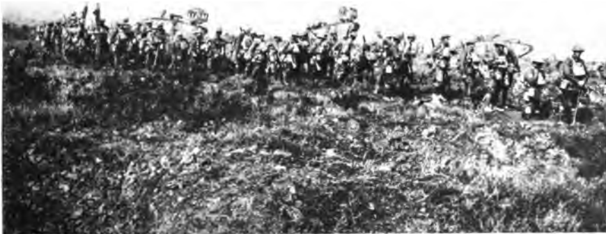
FOLLOWING THE TANKS INTO POSITION
